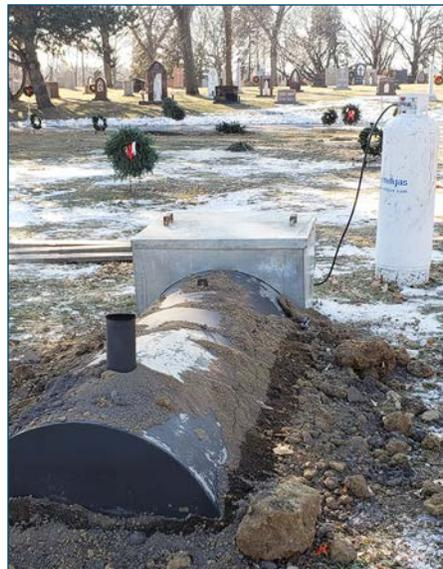
Heat created by a metal hood that is connected to a 100-gallon tank of propane, thaws the earth for winter burials.
